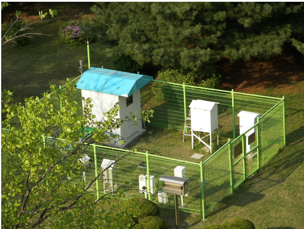
Fig. 2.4 A monitoring post on regional radiation monitoring station
